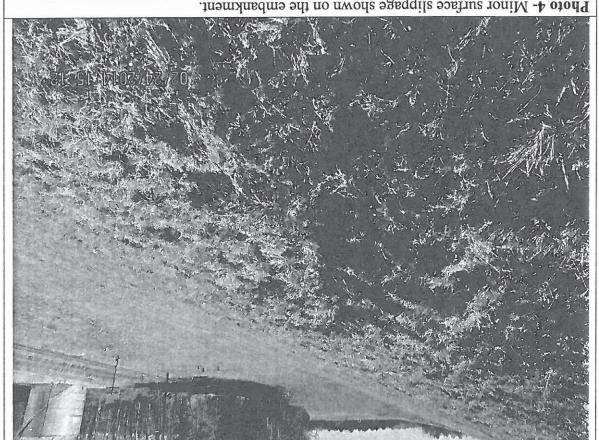
Photo 4- Minor surface slippage shown on the embankment.
